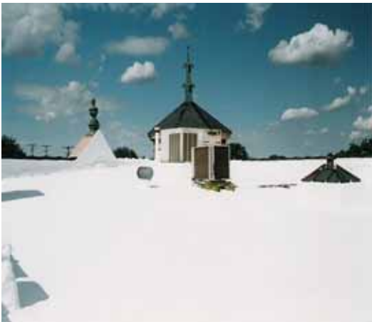
Adurel over built-up asphalt with walls and copings.
