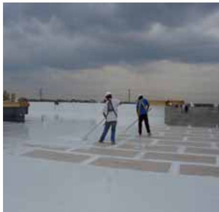
Poured in place seamless technology lowers costs for new construction.
