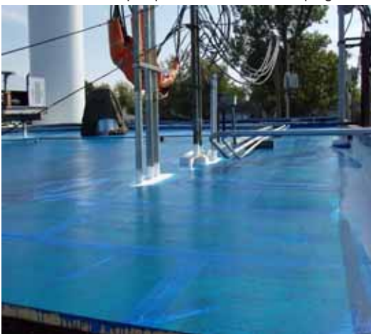
System in progress with resin sealer.
